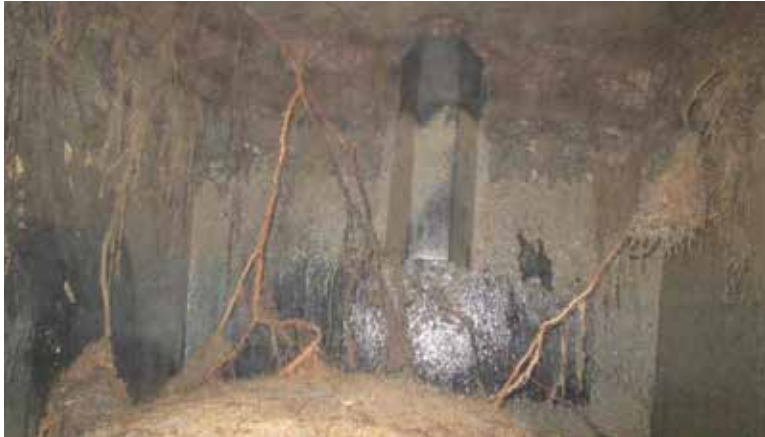
Roots have invaded this tank and are poised to create problems for the septic system.
