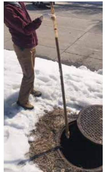
▲ This core sample shows a tank with substantial sludge buildup requiring a pumping service.
