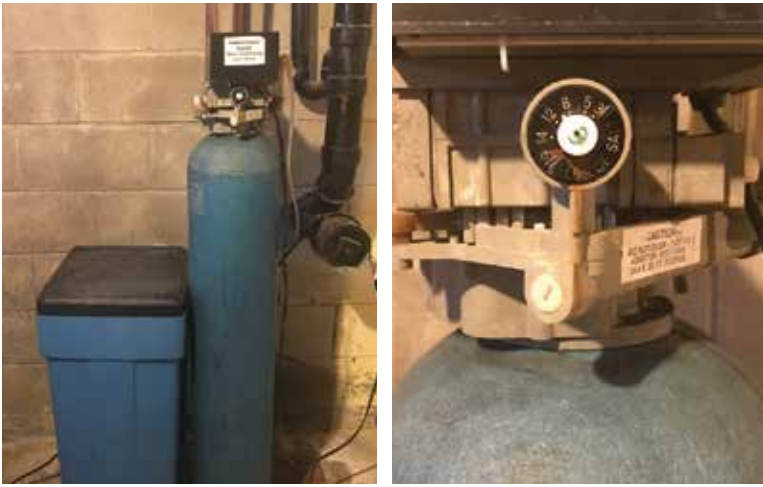
▲ This is an example of the old technology timer-style water softener. The mechanical dial indicates an older timer-style softener.
