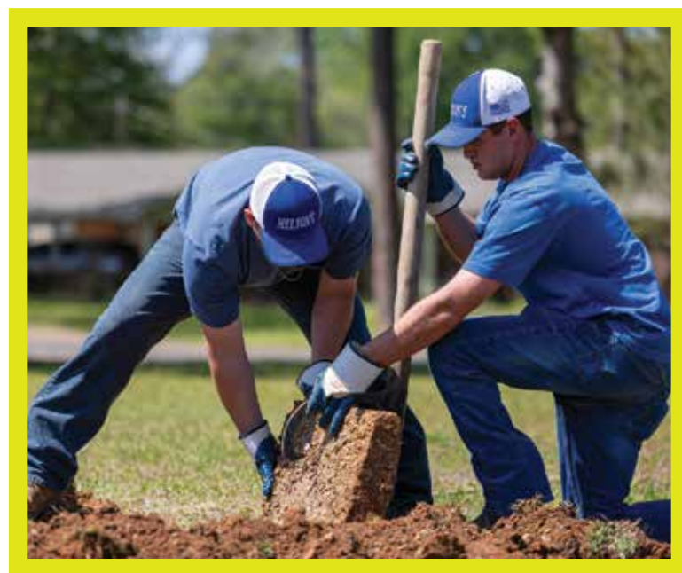
Long and Cooper remove the lid of a septic tank before pumping.
