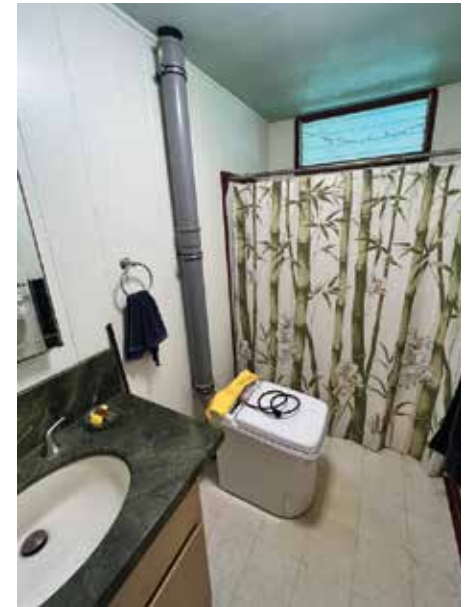
▲ The Cinderella toilet after installation at the house in Kapa'a, Hawaii. The toilet uses electricity to reduce solid waste to ash and evaporates urine. Vapor is vented through the exhaust stack.
