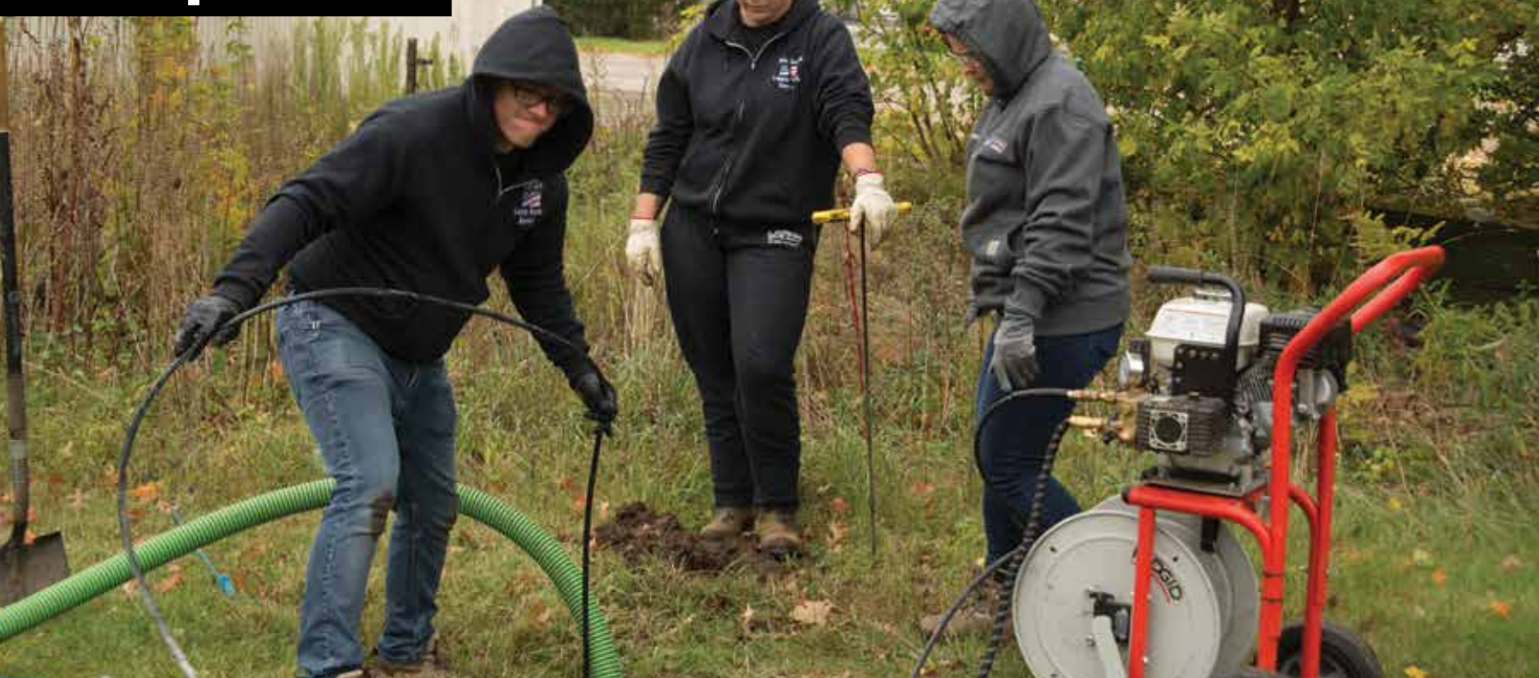
▶ From left, Ben Lappin, Mackenzie Stephenson and Jessica Lappin work with a RIDGID jetter at a residential septic maintenance job.
