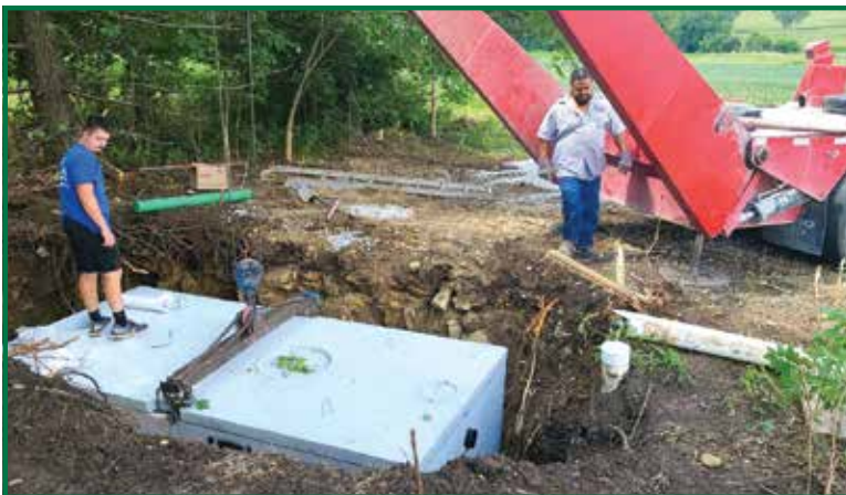
Clint and Bryson McCammon installing an Allied Concrete Products tank.
