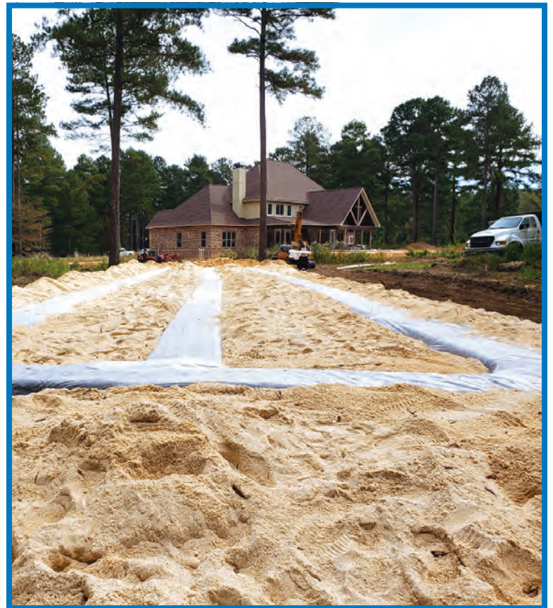
⬆ An ADS Septic Stack in-ground system in a level configuration.
