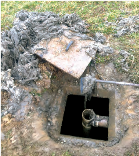
Danny Duncan shared job site photos of the wipes issues he encountered during a recent pumpout. Maybe if customers saw what wipes were doing to their septic systems, they would stop using them.
