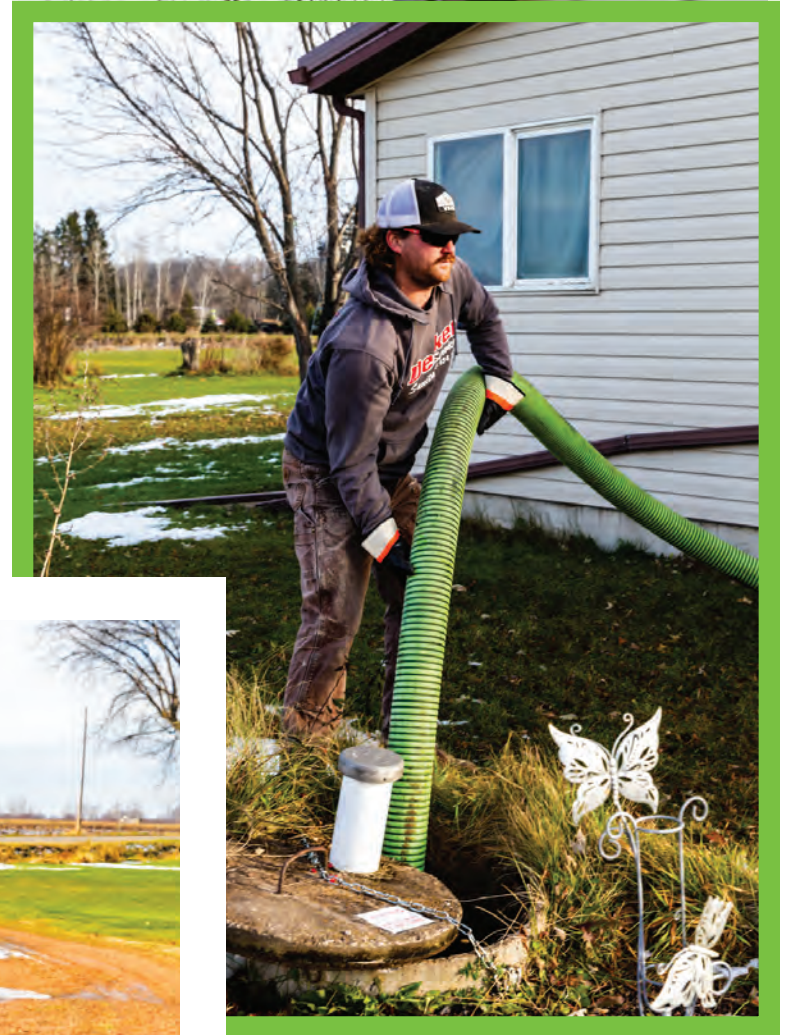
Stickney pumps a residential holding tank. Because of poor soils, the company has more customers on holding tanks than septic systems. The average holding tank holds 4,000 gallons and is pumped every six weeks.
