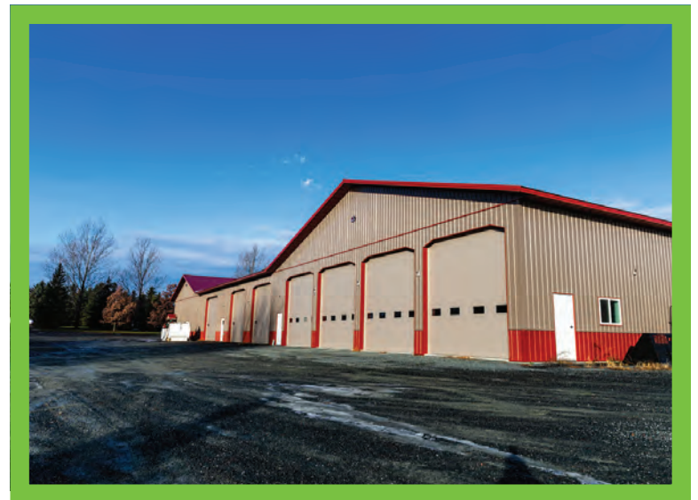
▲ The Decker Sanitation Services shop is set up for year-round equipment maintenance with several bays to keep the trucks out of the harsh Wisconsin weather.
