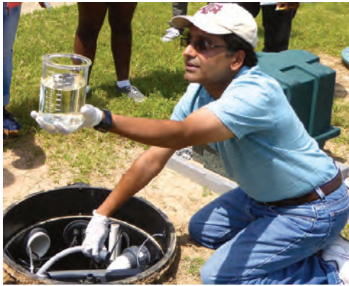
▲ Anish Jantrania, associate professor and extension specialist at Texas A&M University, holds up a beaker of water from an onsite system during an event at the university's On-Site Sewage Facility.
