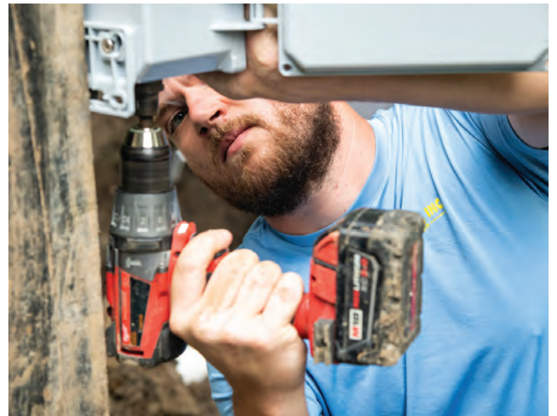
Technician Link installs a control panel box from BioMicrobics.
