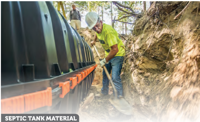
SEPTIC TANK MATERIAL
