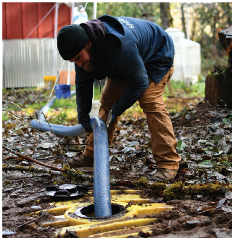
Matthew Peacock pumps graywater from a customer’s 350-gallon holding tank. (Photo by Tyler Gordon)
