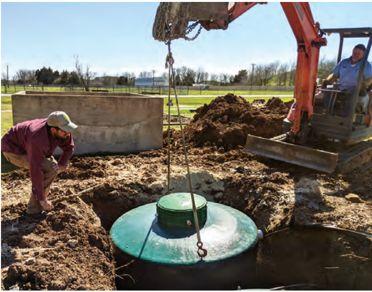
▶ Eric Bob working on an installation of Solar Air tanks for an executive retreat.
