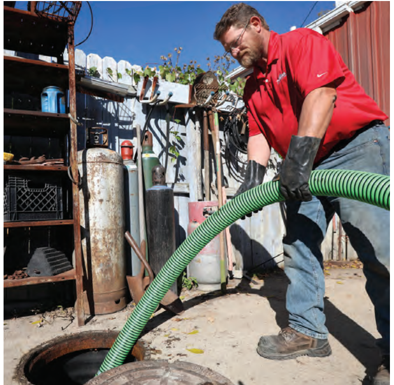
◀ Don Siegers pumps a septic tank at a commercial property in Lake Orion, Michigan.
