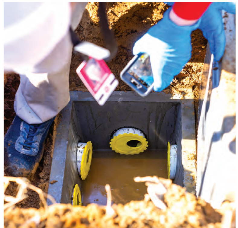
Left: Keith Whitley, left, and Kaine Stephen dig up a septic tank and D-box in a residential system.
