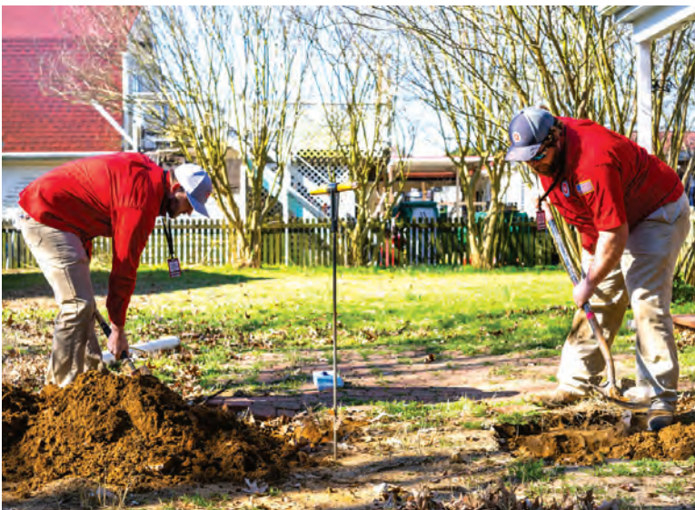
Left: Keith Whitley, left, and Kaine Stephen dig up a septic tank and D-box in a residential system.
