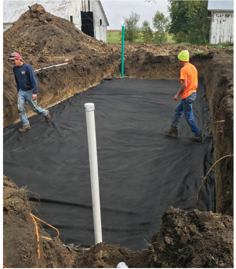
Left: Terry Lunsford and a Wilkinson Heavy Precast 1,500-gallon, three-compartment tank with a pump chamber. Above: Terry and Walker Lunsford cover lines with fabric before laying down sand for a sand-bed secondary treatment system. Below: The Leichy & Son team includes, from left, Terry Lunsford, Micah Johnson, Matt Stalder, Jeremy Farley, Jake Sanow, Walker Lunsford, Steve Davis, Irvin Leichy and Kurt Leichy.
