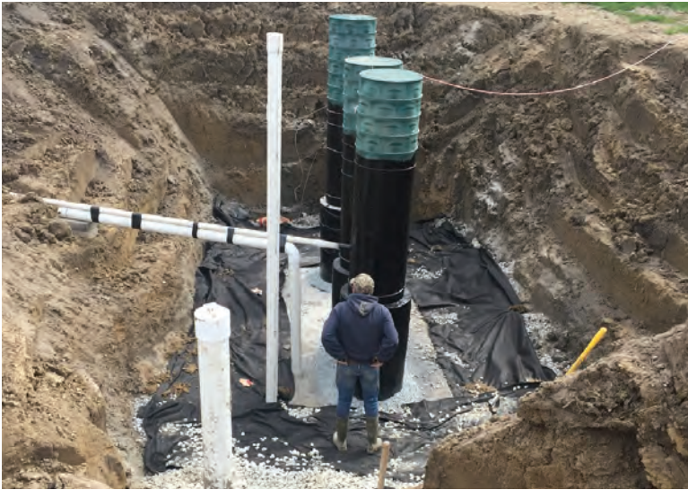
Left: Terry Lunsford and a Wilkinson Heavy Precast 1,500-gallon, three-compartment tank with a pump chamber. Above: Terry and Walker Lunsford cover lines with fabric before laying down sand for a sand-bed secondary treatment system. Below: The Leichy & Son team includes, from left, Terry Lunsford, Micah Johnson, Matt Stalder, Jeremy Farley, Jake Sanow, Walker Lunsford, Steve Davis, Irvin Leichy and Kurt Leichy.
