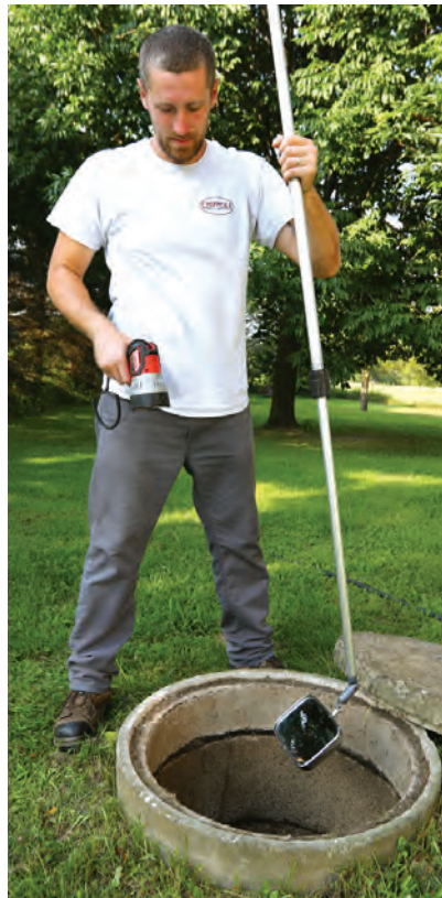
Right: Travis Simet uses a Milwaukee Tool flashlight and a mirror mounted on an extendable pole to inspect the condition of a concrete tank after a pumpout.
