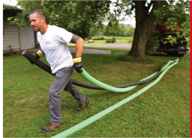
Below: Simet drags hoses to pump a residential septic tank near Eau Claire, Wisconsin.
