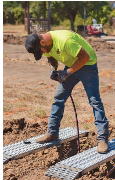
Left: O'Reilly works with driplines in a trench.
