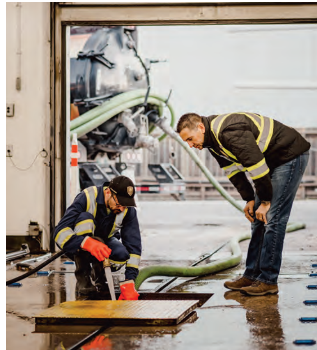
Below: Sizonenka, left, and Steve Moon pump a car wash pit in Winnipeg, Manitoba.
