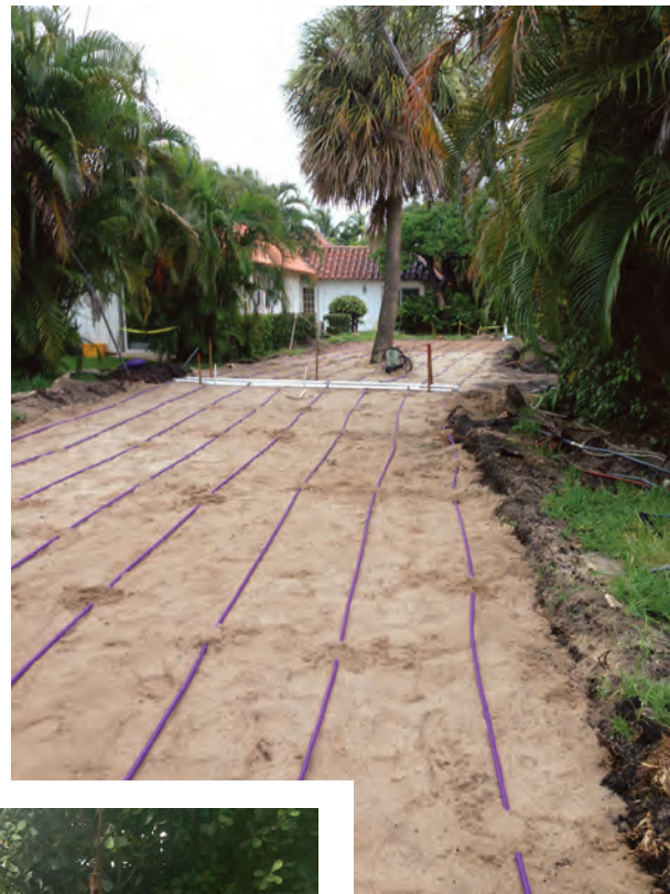
Above: A Netafim dripline is laid out with a BioMicrobics treatment system. Lots in Florida can be tight and systems complex.
