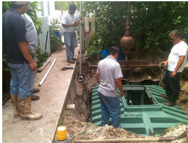
Above: A Netafim dripline is laid out with a BioMicrobics treatment system. Lots in Florida can be tight and systems complex.
