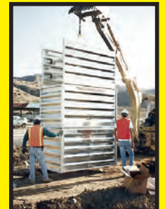
Stacks easily with 2' & 4' high panels.
