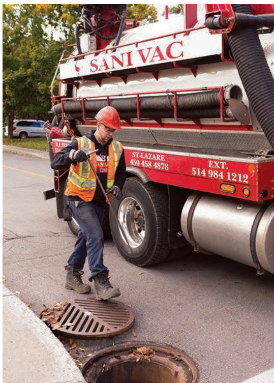
Below: Technician Martin L'Heureux prepares to clean a storm sewer. The truck was built out by Transway Systems and carries a Robuschi blower.
