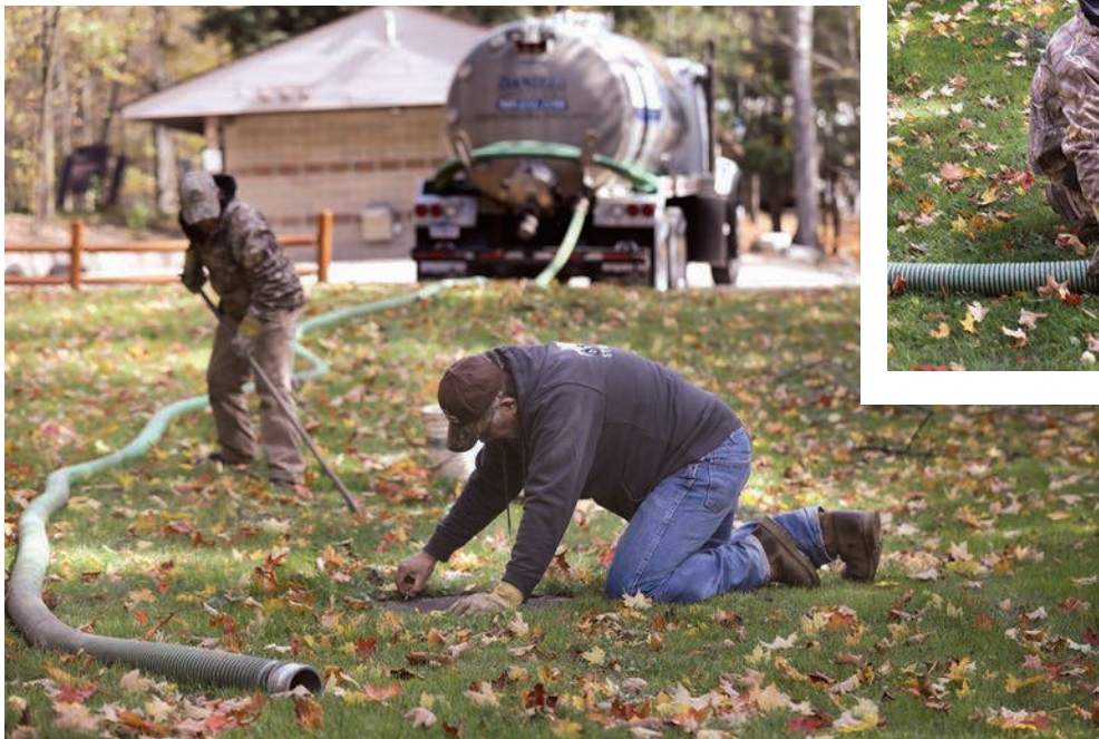
Above: Raymond Daniels probes to locate the access lid on a tank at a residential septic system.
