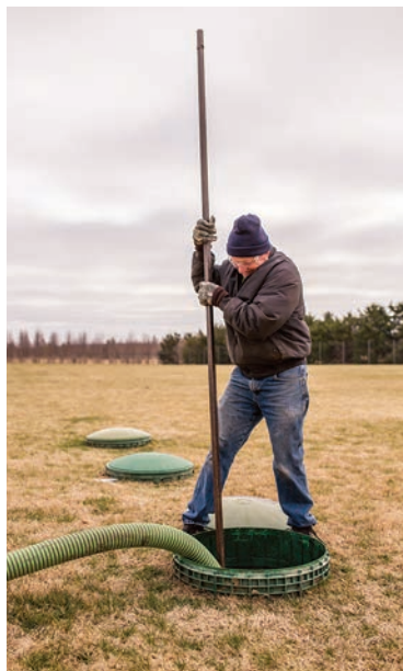
Right: Raymond Smith uses a pole to agitate a tank during a pumping job. The system uses TUF-TITE risers and lids.
