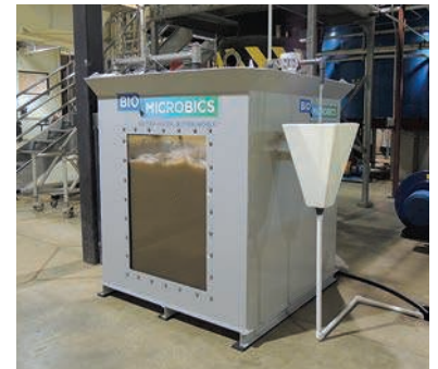
Above: Up and running, the new membrane bioreactor at Southern Illinois University Edwardsville has become part of the equipment used to train new wastewater equipment operators and to provide continuing education for licensed operators. MBRs have been used in onsite installations for some time and are also being more widely used in municipal wastewater plants.
