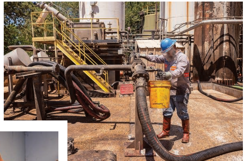
Above: Jose Chavez operates an off-loading valve as he empties a tanker.
