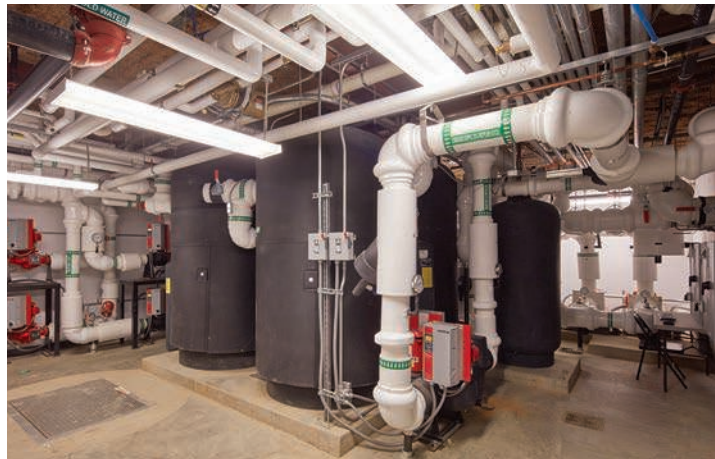
Left: The TSE (treated sanitary effluent) Treatment room includes pumps (left) from Grundfos Pumps that convey treated water from a storage tank to toilets throughout the building for use in flushing.
