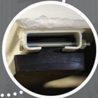
rubber t-track mount stainless channel
