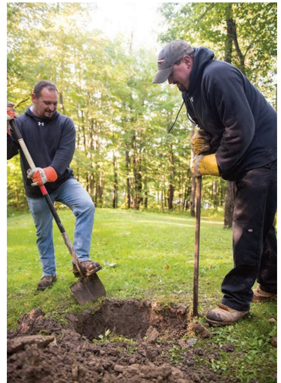
Above: Moe Kurowski, left, and Vinnie Zuech dig to locate a lid while serving a residential septic system.
