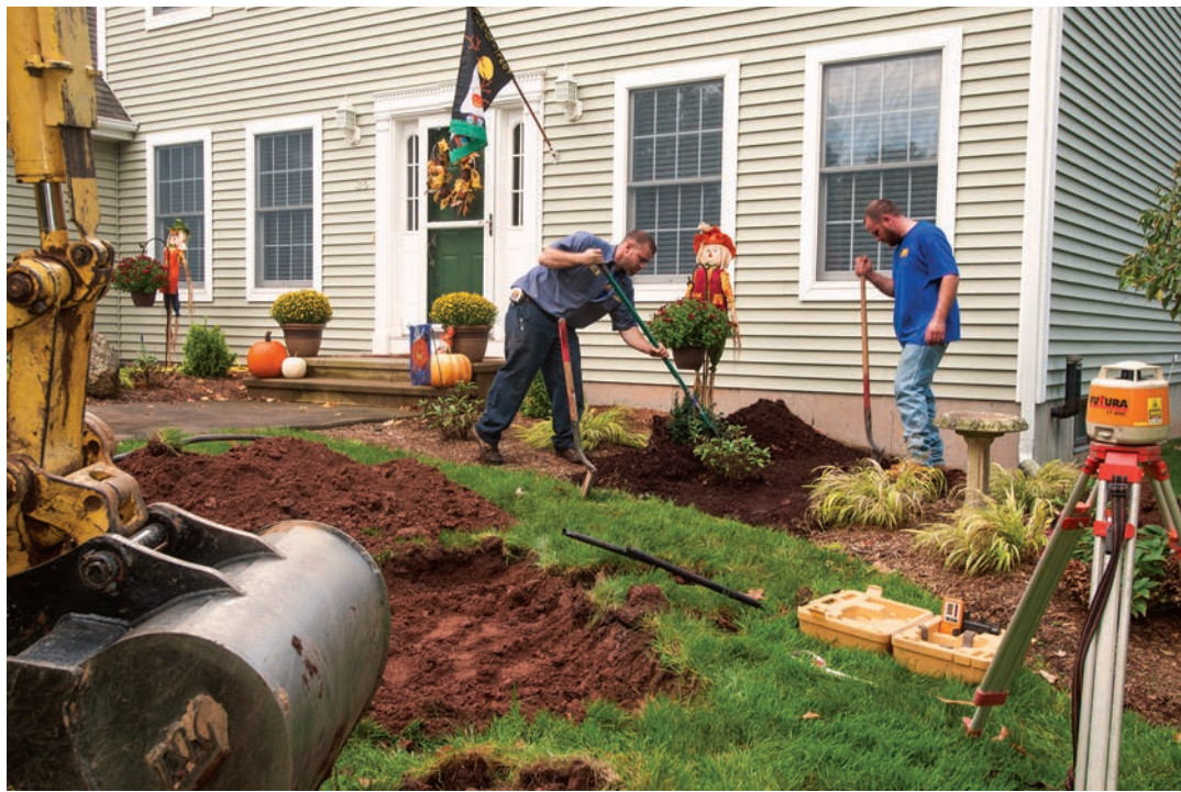
Left: Justin Breault and Matt Choptij dig a trench through a garden bed for a water softener discharge drywell. They are using a Futura LT-800 laser level.
