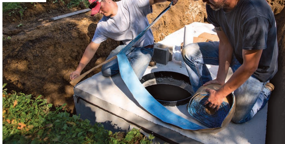
Right: Dylan Jacobs, left, and Anthony Schmitz seal a concrete tank lid during a septic system installation.
