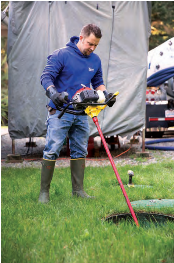
Left: Shawn Carlton utilizes a Crust Buster tank agitator to break up the contents of a customer's full septic tank.
