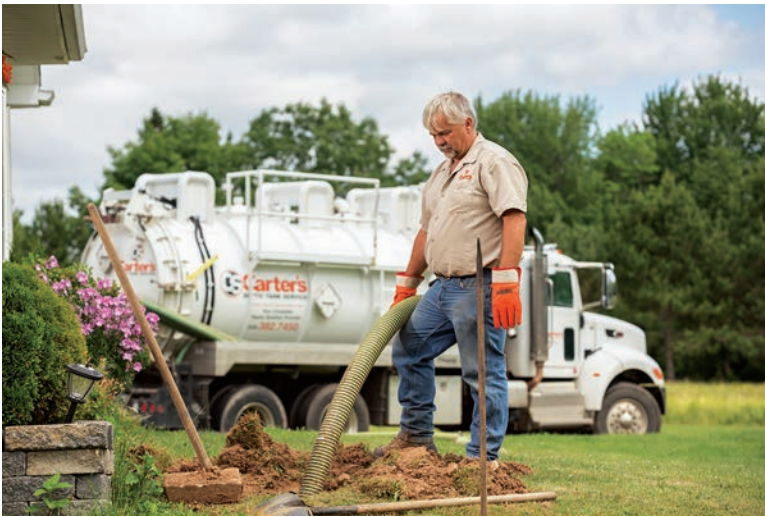
Brad Carter pumps a septic tank using a Peterbilt vacuum truck built out by Imperial Industries with a Fruitland pump.
