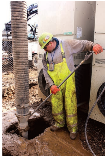
Left: Schmoll works in tight quarters with a Premier hydroexcavator.
