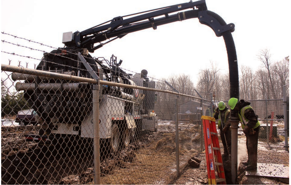
Left: Schmoll works in tight quarters with a Premier hydroexcavator.
