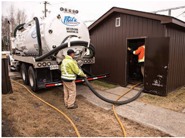
Right: Technician Stephen Gillespie (holding the hose) and an unidentified municipal worker clean a lift station using the company's Sterling vacuum truck with a Fruitland pump and built out by SchellVac Equipment.
