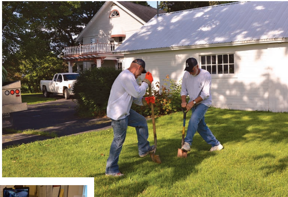
Right: Jason Miller and Terry Fiedler use shovels to uncover a septic tank lid during a residential service job.
