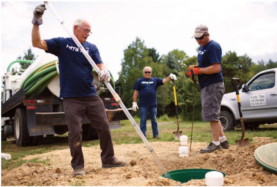
Left: Dave Hess uses a Sludge Judge (Nasco) while Darrell Swatsworth and Scott Hess check out a recently completed septic tank repair for a Pennsylvania Septage Management Association final inspection.
