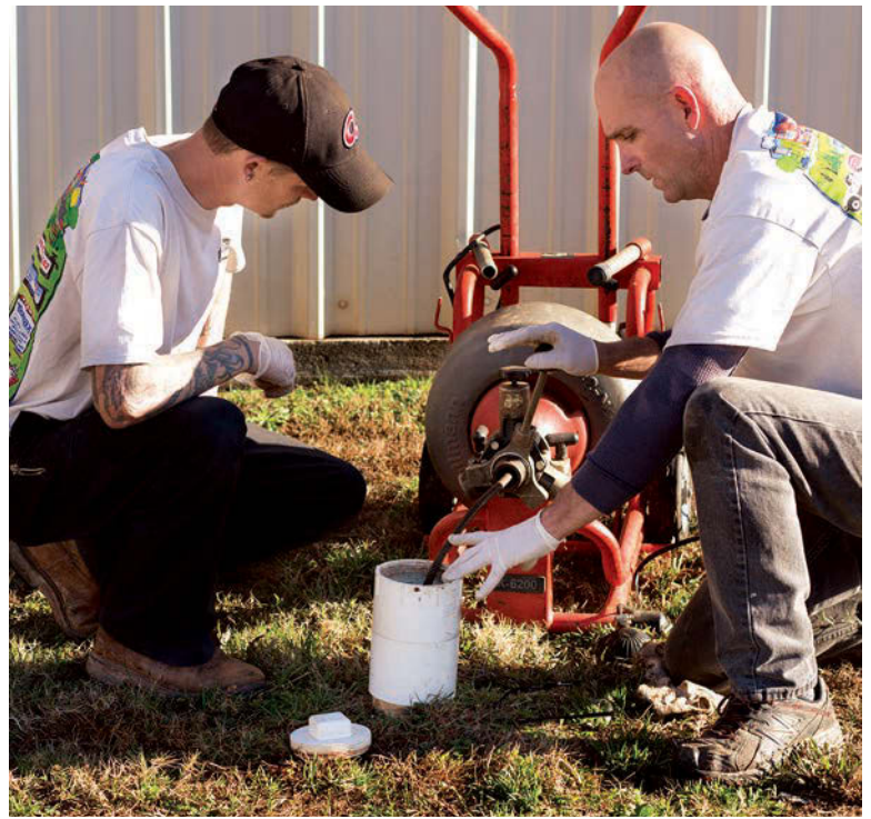
Above: James Brooks, left, and Todd Davis use a RIDGID K-6200 drum machine during a service call.
