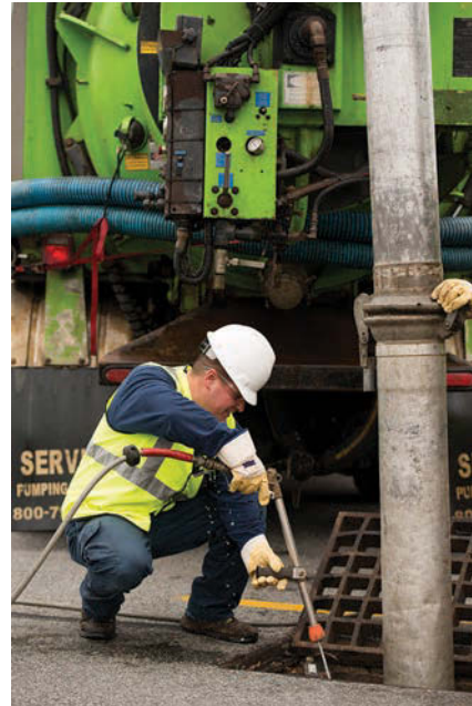
Technician John Perry cleans out a catch basin using an Aquatech B-10 combination unit.
