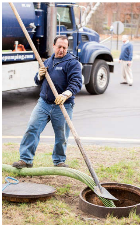
Left: Technician Janio Storck pumps a hotel holding tank using a service truck from Andert with a 4,000-gallon tank and National Vacuum Equipment pump.
