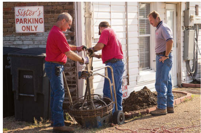
Below: Mark Vice, right, watches as Jeff Goree and Josh Jackson clear a drain at a local business using a Duracable Manufacturing Co. drain cleaning machine.
