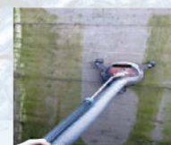
Air Recovery Works on Walls
