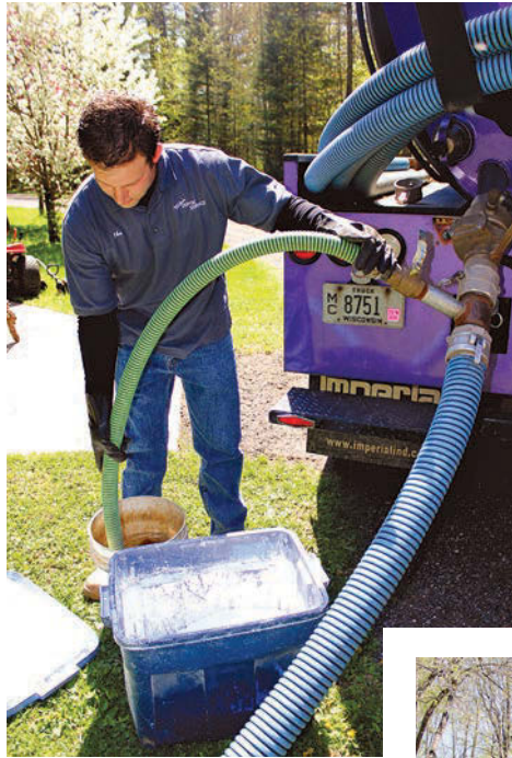
Left: Technician Ike Roberts adds lime to the tank during a pumping job.
