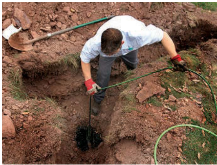
Mounted below his truck's hose tray, a toolbox jetter from Advance Pump & Equipment comes in handy to clear a clogged line during a maintenance call.
