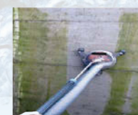
Air Recovery Works on Walls
