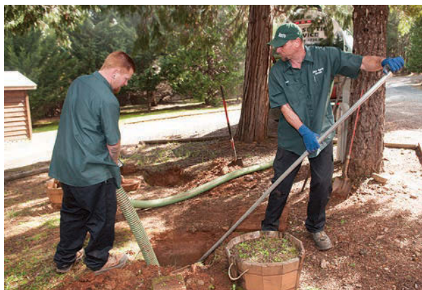
Below: Technician Doug Modgling controls the hose, while Fiske uses a custom-made 10-foot aluminum rake to keep the slurry moving during a pumpout. The rake has a 3/8-inch-thick aluminum plate welded to the working end.
