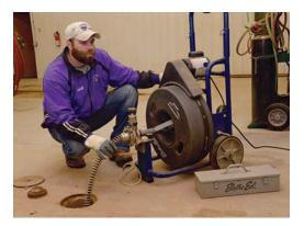
Ardell Kick uses an Electric Eel machine to clear a customer's floor drain.
