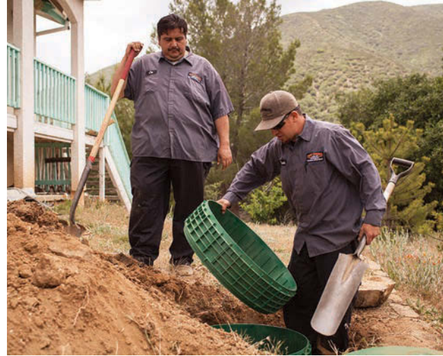
Below: Medina and Herrera install Tuf-Tite risers to make for easier future access to a customer's septic tank.
