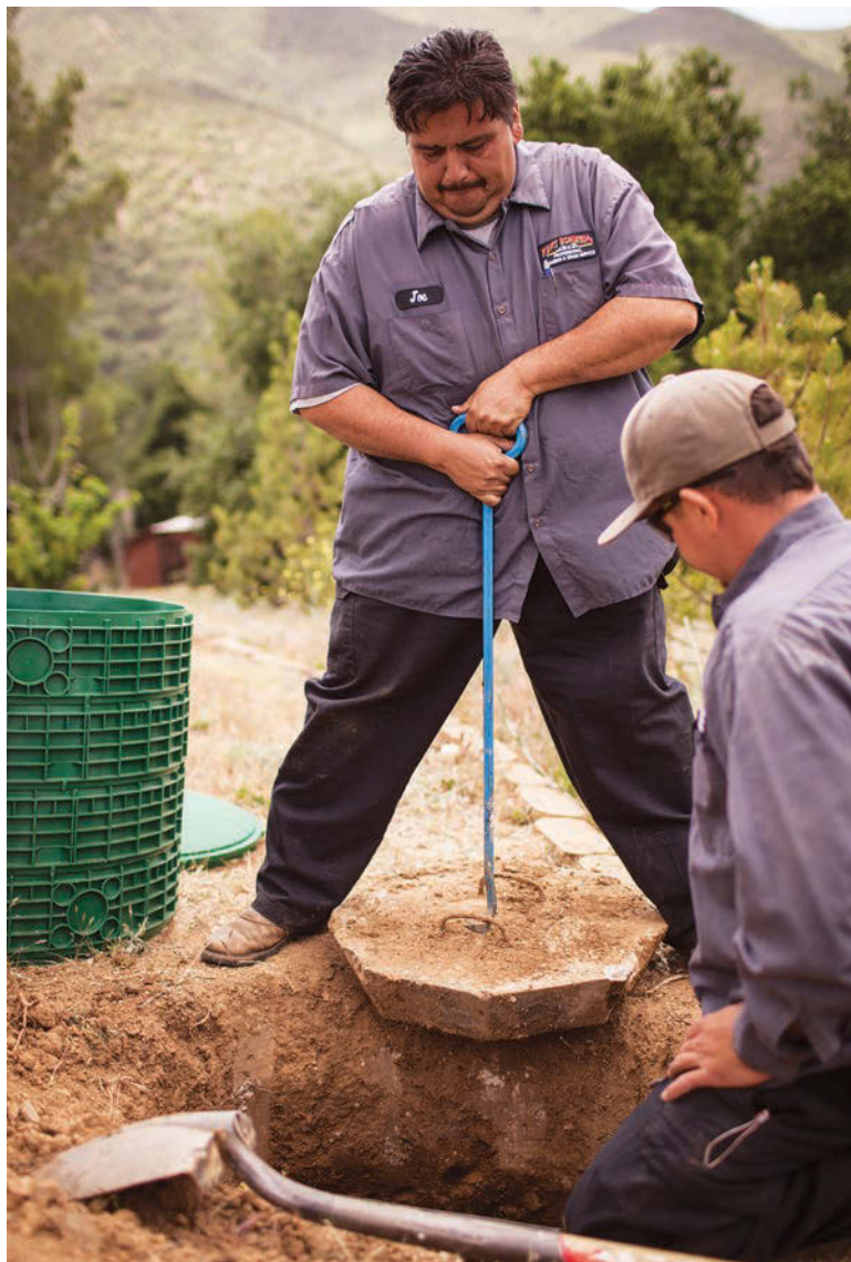
Left: Employee Joe Medina pulls a concrete tank lid using a Top Popper from T&T Tools, Inc. as Eusevio Herrera looks on.
