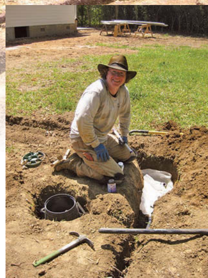
Philip McCreanor, associate professor at Mercer University, installs one of the corner connections of a dripline at a Habitat for Humanity house in Macon, Ga.
