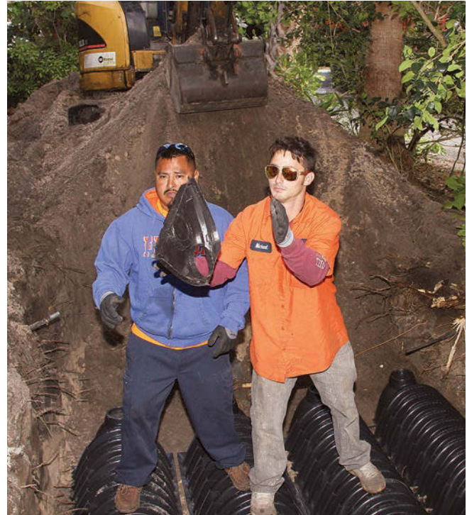
Below: Installers Ramon Santiago (left) and Michael Ruehman place an Infiltrator Systems chamber as part of a new septic system in Indian River Shores, Fla.
