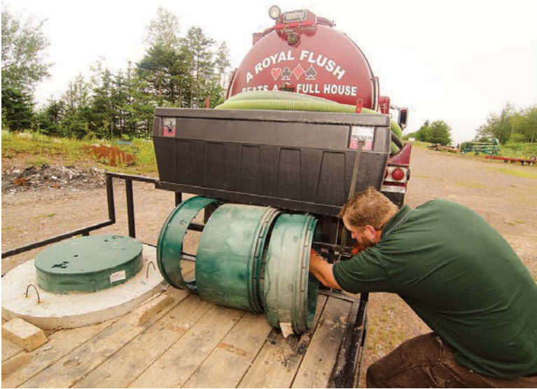
Left: Bio-Liquid Waste Disposal encourages homeowners to install risers and lids to systems for more convenient pumping and inspection. Andy Ledrew is shown loading a truck for delivery.
