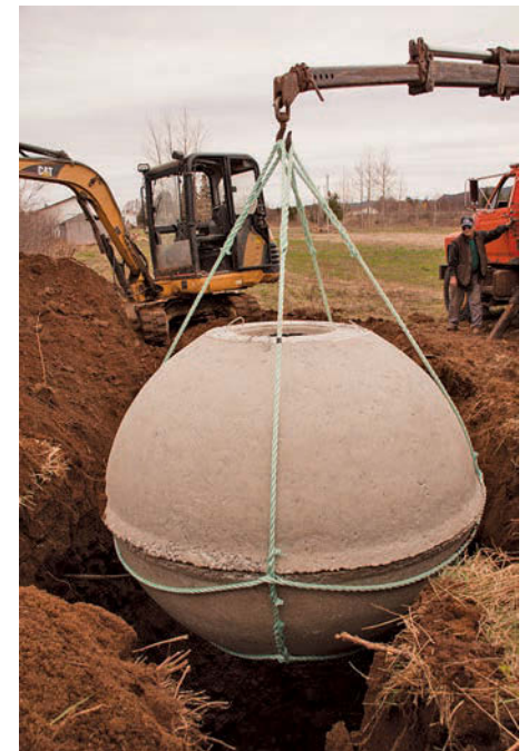
Below: Gerard Gale stands by the boom truck while a new Turtle Tank is lowered into the ground.
