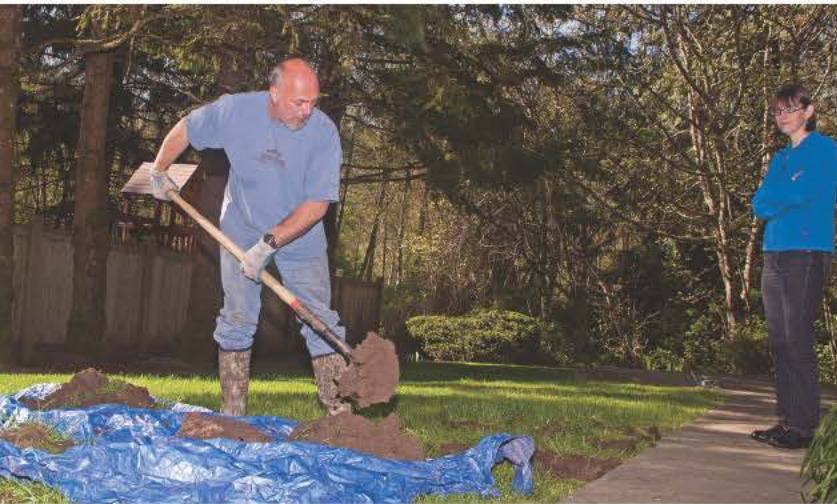
Above: Margaret Rosenberg, a regular customer, looks on as Long exposes her tank lid during a pumping job. Long shovels dirt onto a tarp to limit the mess.
