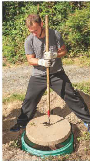
Cory Couty removes the lid from a septic tank.
