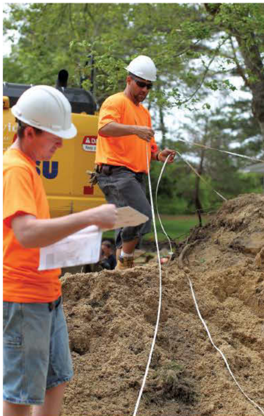
Technician Marvin Meyer works on the installation of a 1,000-gallon septic tank as part of a new onsite system. >>>
